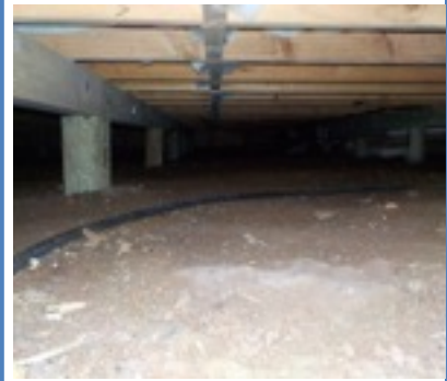
Figure 2:subfloor is in good condition and is insulated and dry.
